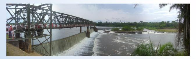
Situation in March 2008 during ending of flooding period. The old spillway system was built in the 50s and is no longer safe. In consequence the whole EDEA Hydropower plant and with it the Alucam aluminium factory in Edea as well as the south of Cameroon private consumption is in big danger of huge energy losses. The new modern spillway system will be built 6 m downstream of the old dam axis.
